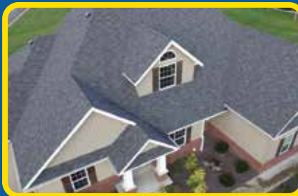
Roofing, Siding, & Gutters
